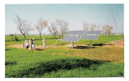
Fig. 12.2 Photovoltaic Water Pumping
